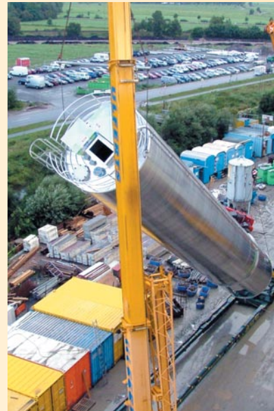
Ill. 1: Starch silos
